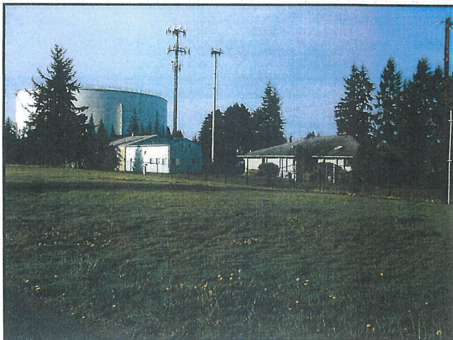
East side of Subject office and shop – view from 132 nd Street SE.
