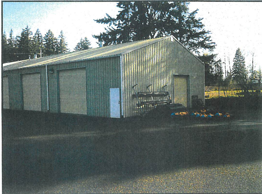
South end of shop/maintenance building.
