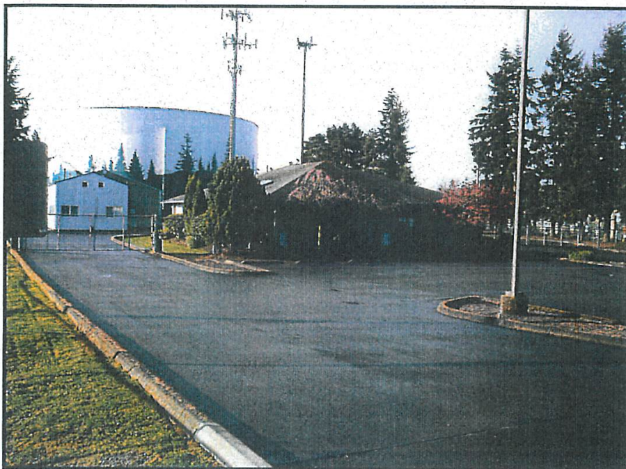
Subject office and shop – view from 132 nd Street SE.
