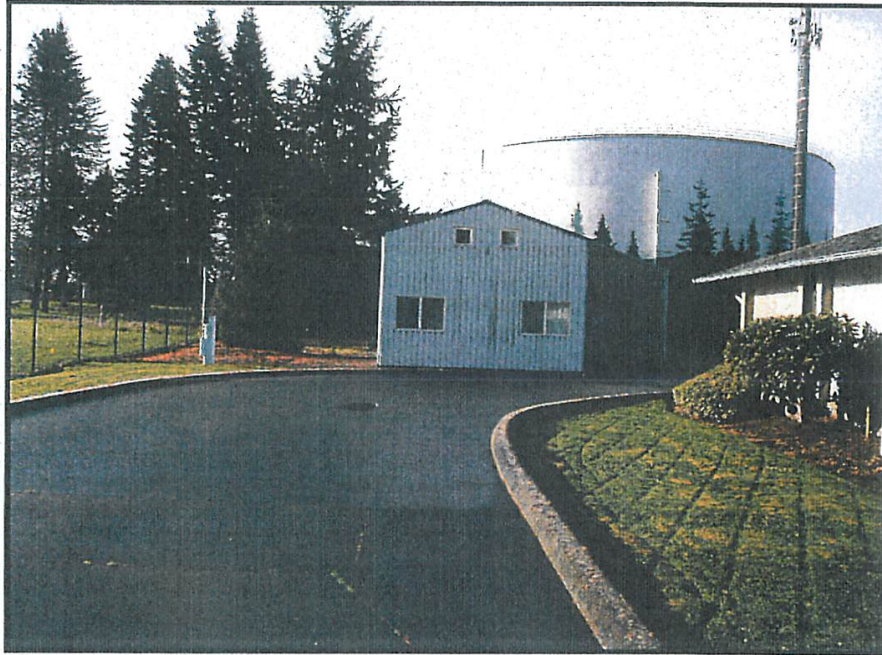
North side of shop building, office on right.
