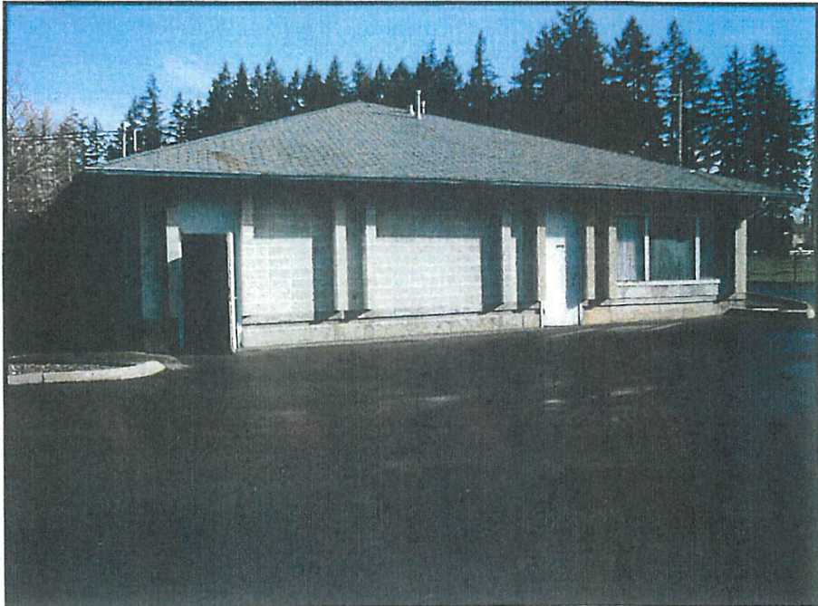
Subject office - rear view.
